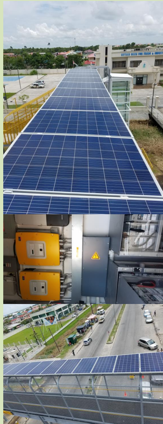
AC Coupled Systems & BESS w/Grid Feed In & Frequency Shifting Capability Installed @ Pedestrian Overpasses EBD
