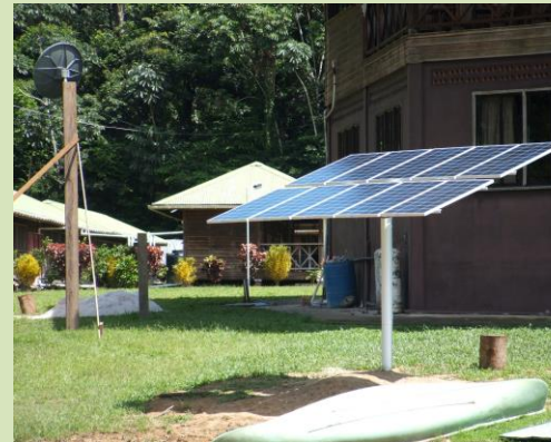
Solar Array Installation @ Iwokrama River Lodge
