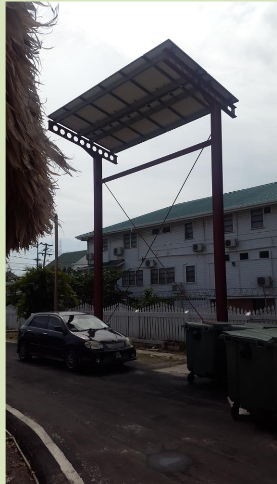
PV Array Installed @ 15m to Clear Shading
