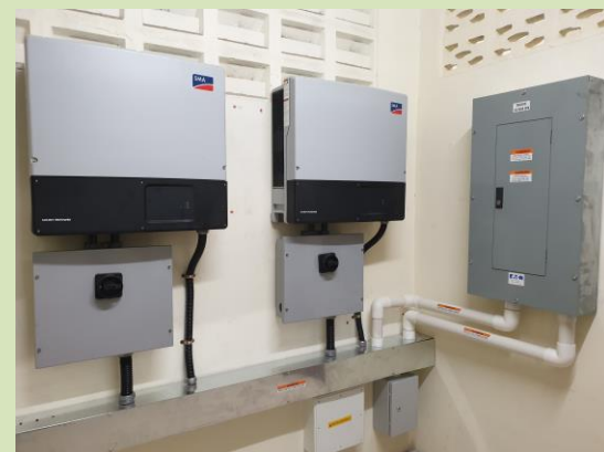
Grid Connected Inverter Installation
